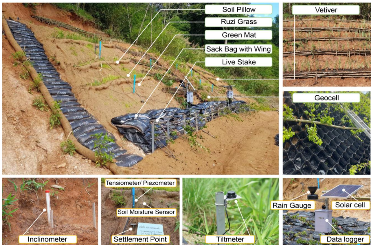
Figure 6 - Photographs of test section 4.
