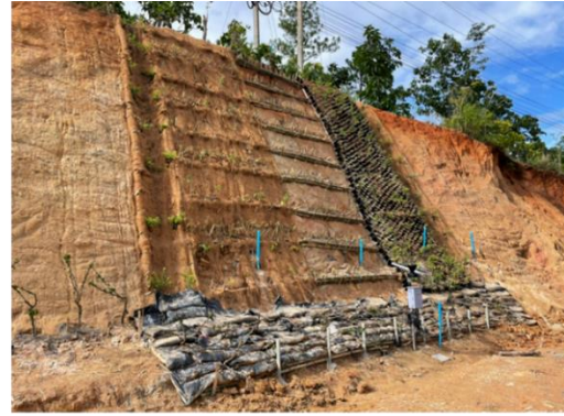
After construction 2022- July
